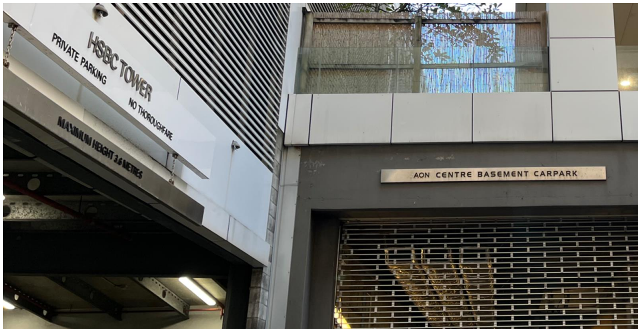
Figure 25: Sign posted vertical clearance restriction of 3.6 m on existing service lane
